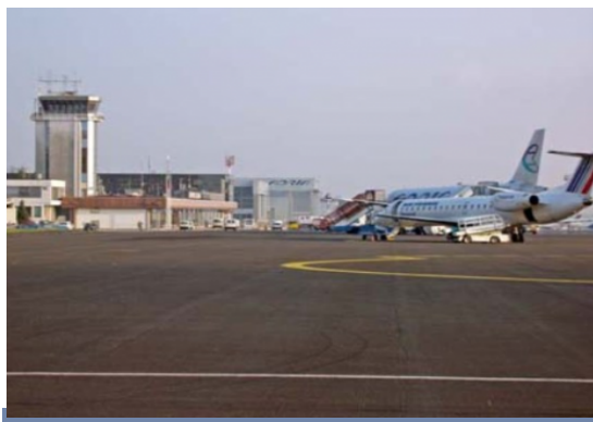
Airport Maribor - ( CCTV, Fire, Access Control, Intrusion, BIS )
