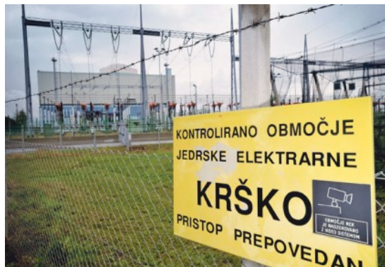
GEN Krško Plant – Krško (Fire alarm, Intrusion)
