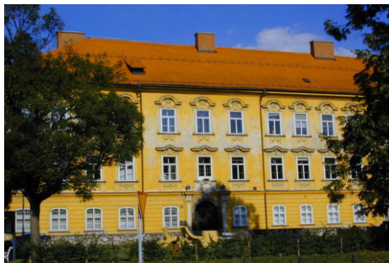
The Archives of the Republic of Slovenia – ( Fire Alarm )
